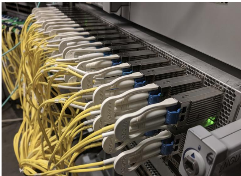
Shown are 36 NeoPhotonics QSFP-DD 400ZR Modules Operating in an Arista Switch
